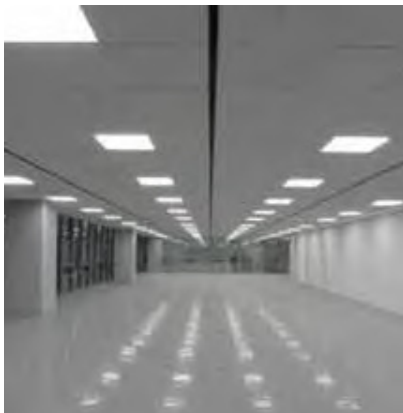
Highly efficient LED lighting
