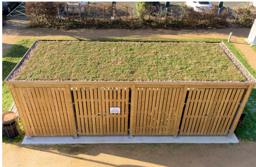
Example of Green Roof Bike Shelter
